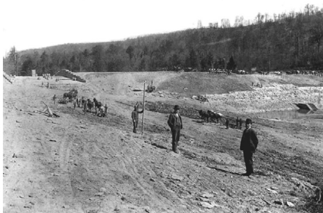
Figure 5 Bradford Dam No.3 (circa 1898) under construction
