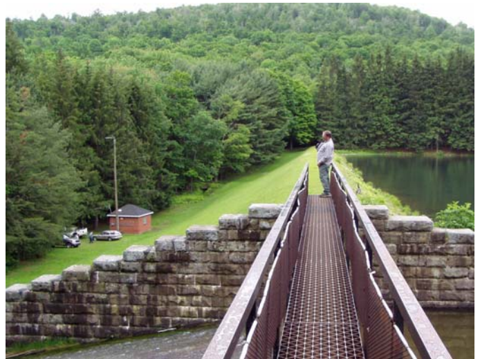
Figure 1 Bradford No.3 Dam at Spillway
